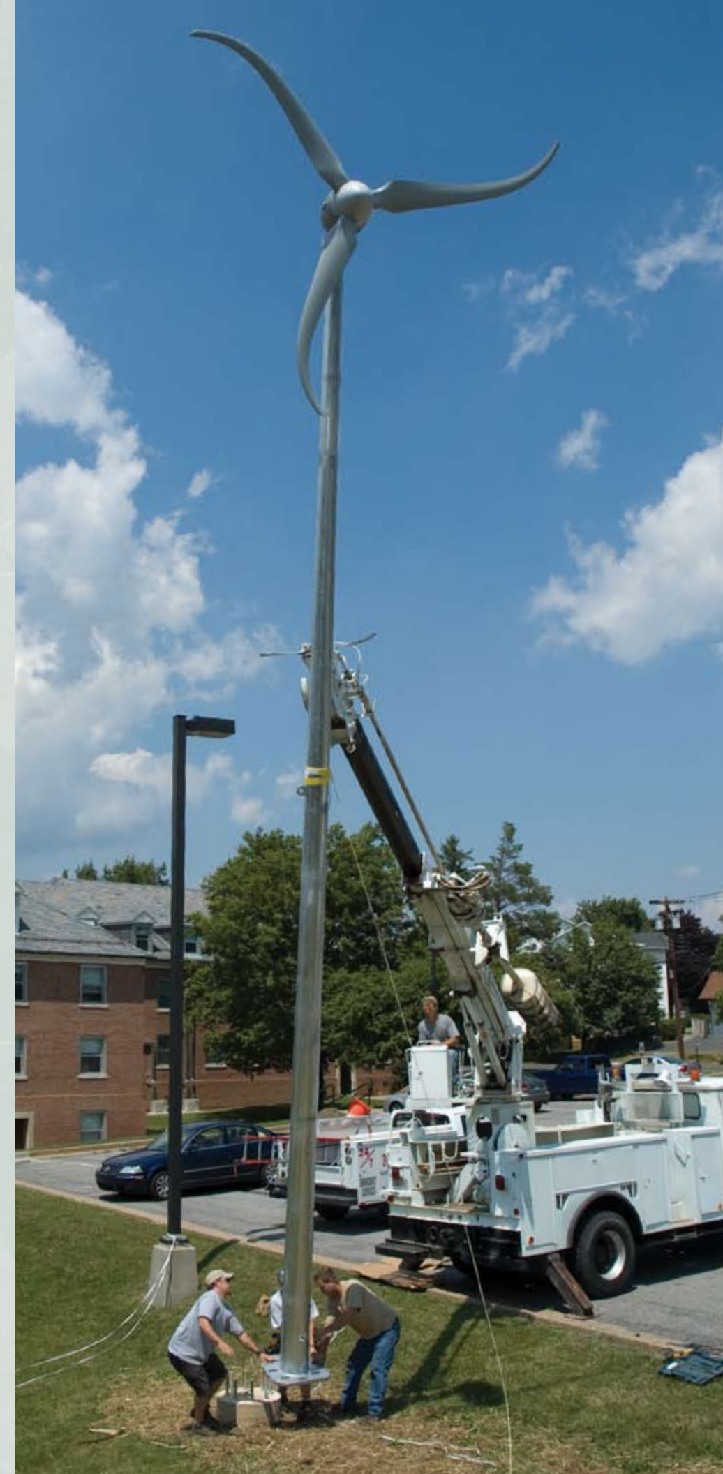
A residential scale wind turbine, part of the WISE project, was erected between the Fuller House and Gray Hall on July 6.
